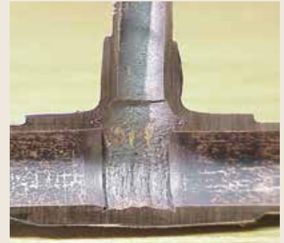
Copper tubing brazed without nitrogen purge. *Notice the black oxide deposits.
